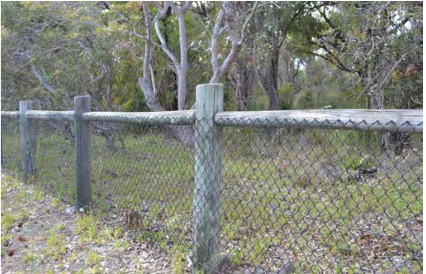
Figure 27: Fencing on the Perimeter of Warwick Open Space
