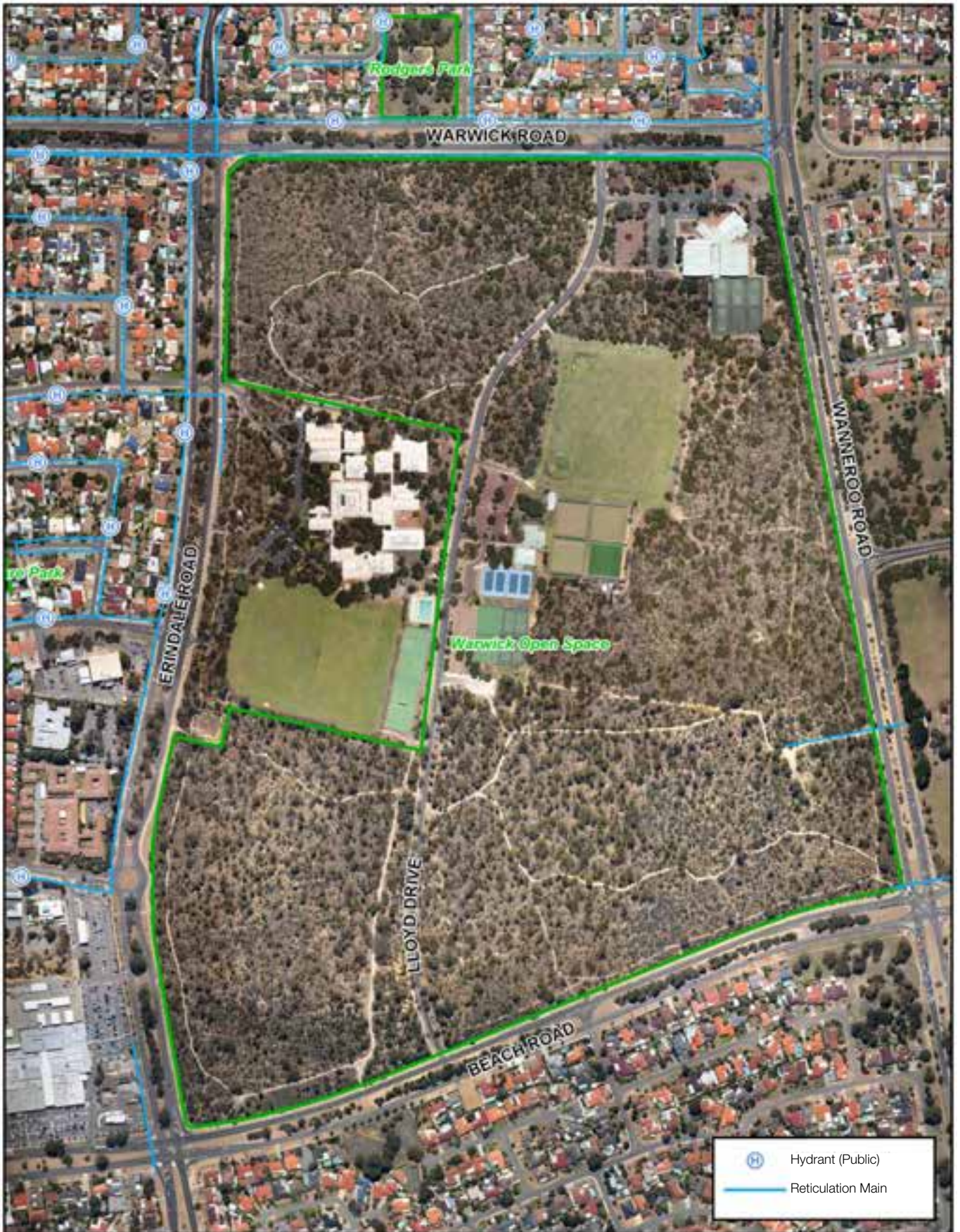
Figure 25: Warwick Open Space Water Utilities
