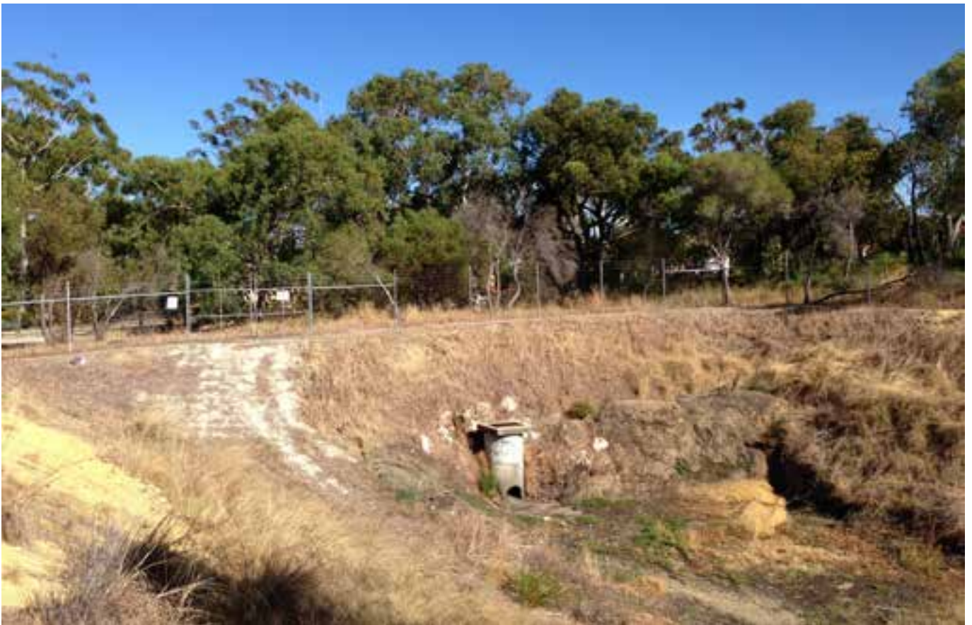
Figure 31: Fenced off Sump at Warwick Open Space
