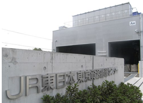
JR East Tokyo Materials Recycling Center
