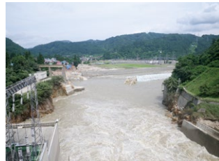
The 6 th Tadami River Bridge
