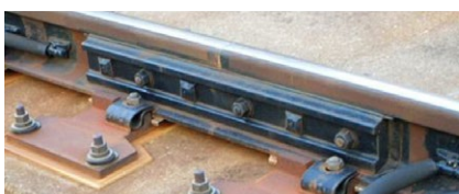
Before improving glued insulated joints
