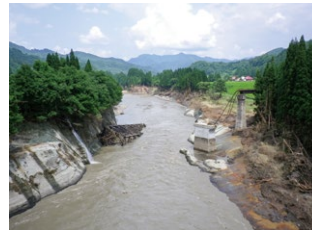
The 7 th Tadami River Bridge
