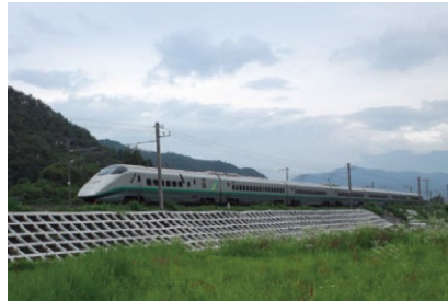
Embankment slope protection (spray frame work)
