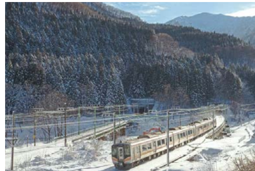
Shigekura No.1 railway forest on the Joetsu Line (forest to protect against snow slides)
