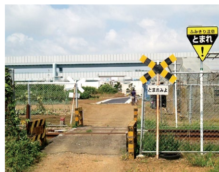
Class 4 level crossing
