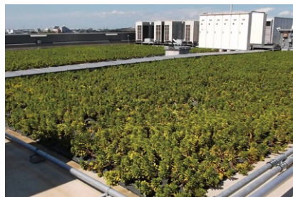
Rooftop greenery at the Chiba branch building
