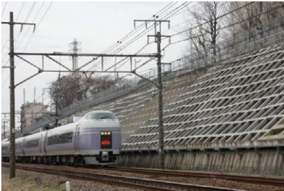
Cutting slope protection (spray frame work)
