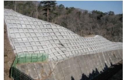
Natural slope protection (spray frame work)
