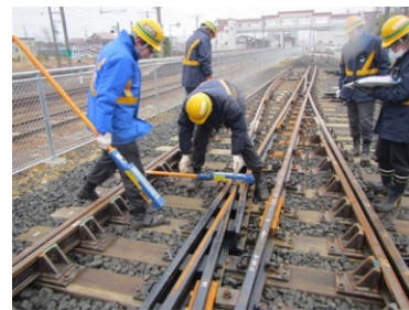
Track facility at Skills Training Center
