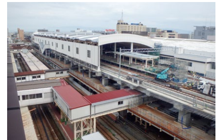
Entire view of Niigata Station
