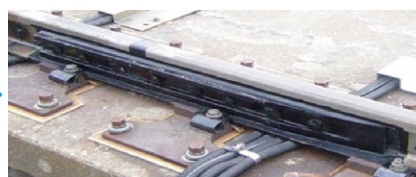
After improving glued insulated joints
