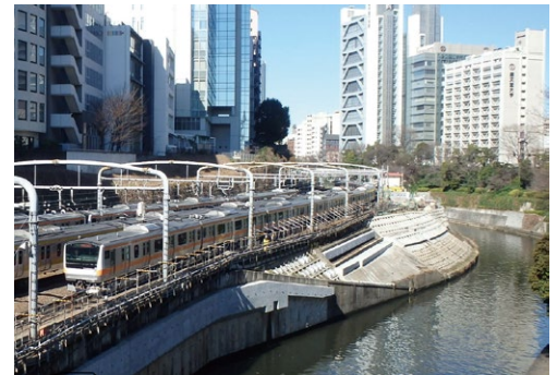
Seismic reinforcement of embankment
