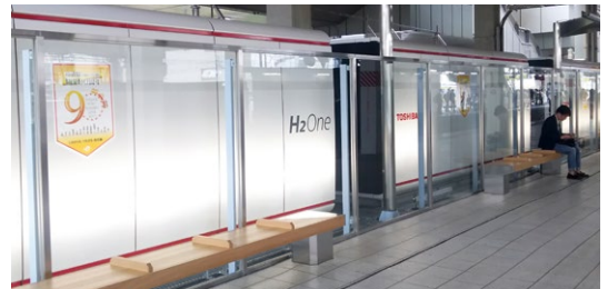
Independent hydrogen energy supply system (Musashi-Mizonokuchi Station)
