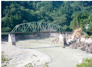
The 5 th Tadami River Bridge
