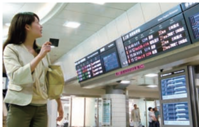
New electronic schedule board installed at Tokyo Station to augment capabilities for flexibly responding to the addition of Shinkansen trains
