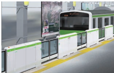
Automatic platform gates
