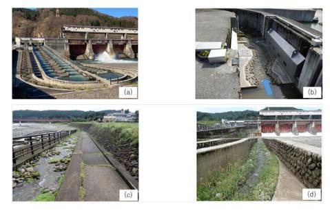
**Figure 1.** Photos of Miyanaka Intake Dam: (**a**) dam and fishway from the downstream side, (**b**) a sector gate at the upstream end of the rock-ramp fishway; the dam end of the sector gate rises by 0.5 m when flooded or when needed for maintenance, the blue arrow indicates the direction of flow, (**c**) rock-ramp fishway and the revetment on the right bank side from the upstream side of the dam, (**d**) the turn-around section of the rock-ramp fishway from the downstream side.
