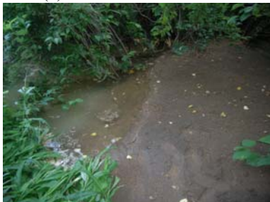
(c)盛土のり先の状況
