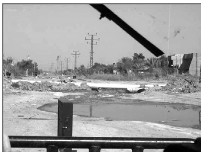
Figure 19. Typical Electric Grid infrastructure in Baghdad
