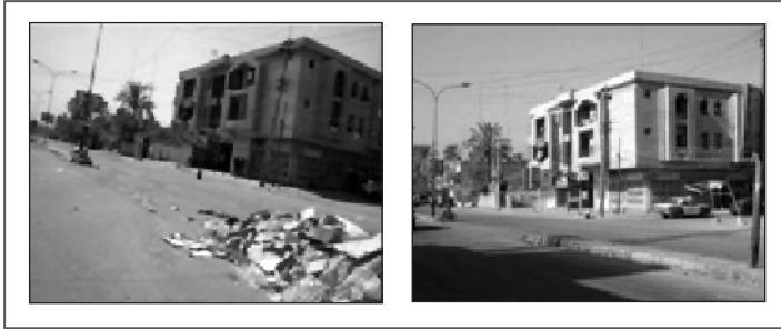
Figure 23. Muhallah 316, before (30 August) and after (6 September)
