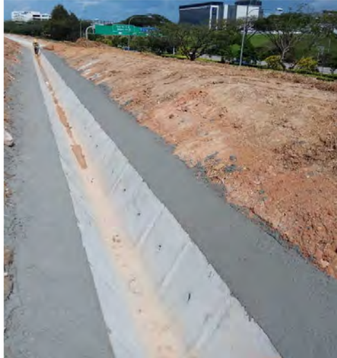
Figure 9: Casting of concrete lining for the C7 drain slope
