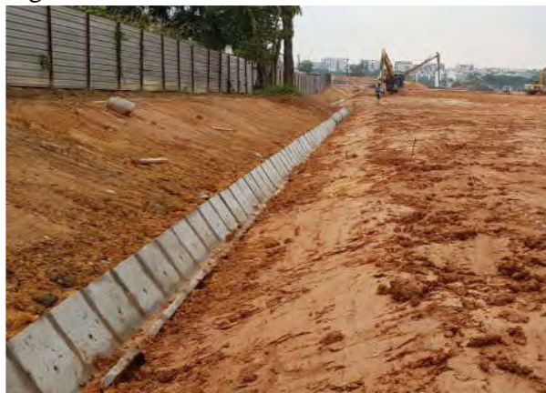
Figure 8: Compaction of slope adjacent to C7 drain
