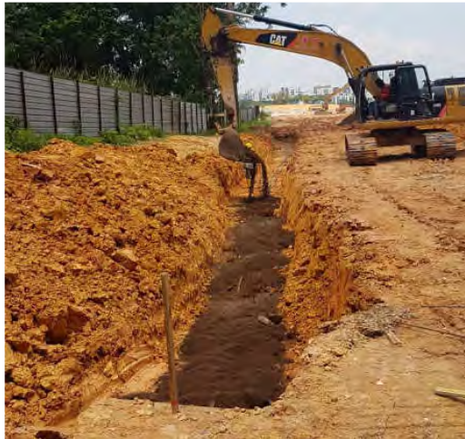
Figure 6: Laying of sand for C7 drain
