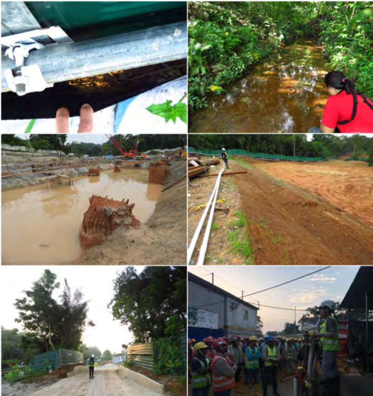
Figure 60: Photographs showing monthly fauna inspections to ensure integrity of hoarding, inspect sensitive habitats in proximity, ensure there is no trapped fauna (e.g., in ECM sedimentation ponds, erosion control blankets), and biodiversity awareness training for site personnel
