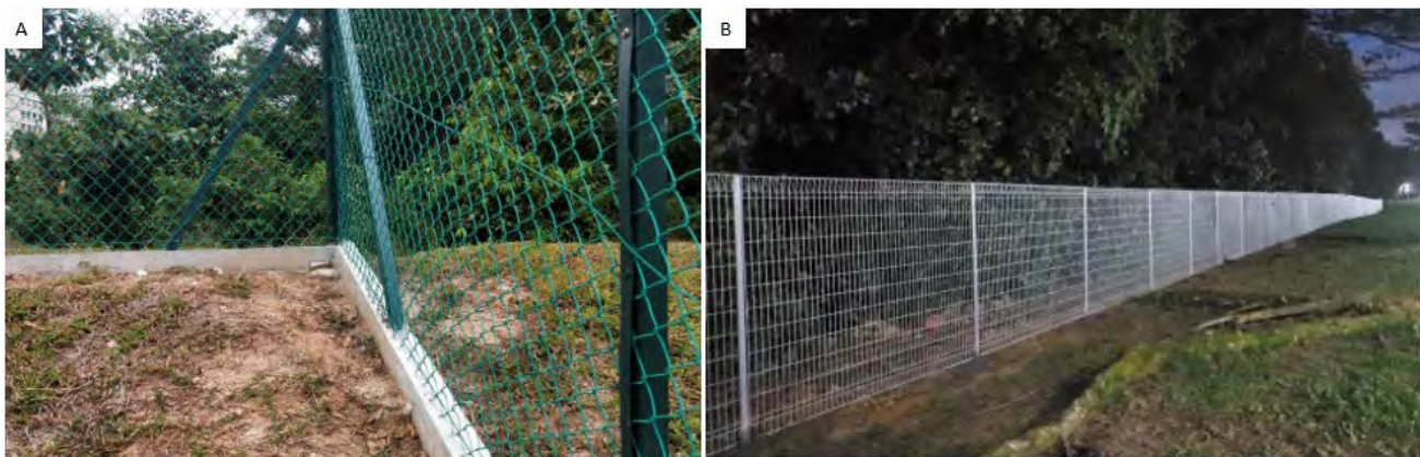
Figure 55: (A) Fences with cement base to prevent animals from burrowing through them; (B) BRC or weldfences along a vegetated area at Pasir Ris Park
