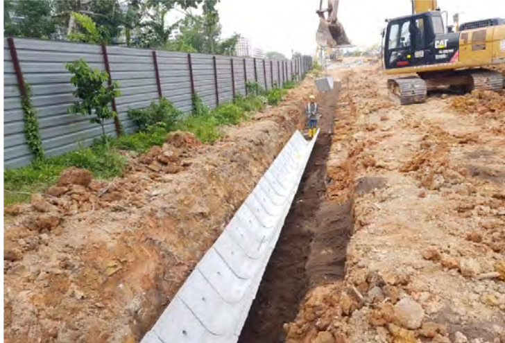
Figure 7: Laying of C7 drain
