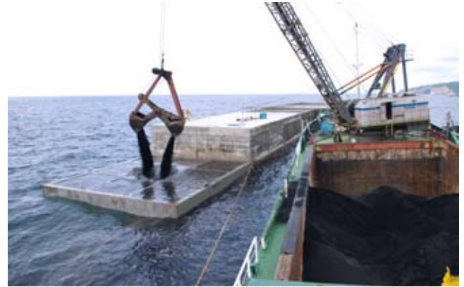
Drop-in operation of iron silicate slag in caissons
