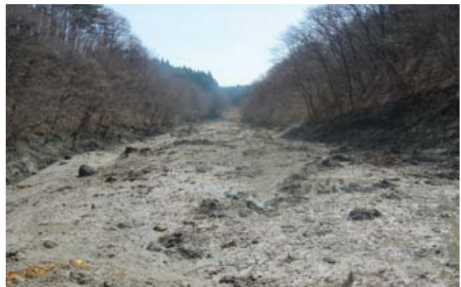
Scene of the outflow of tailings just after the earthquake (April 2011)
