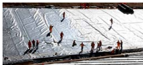
View of operation for the construction of dump leach pad facilities
