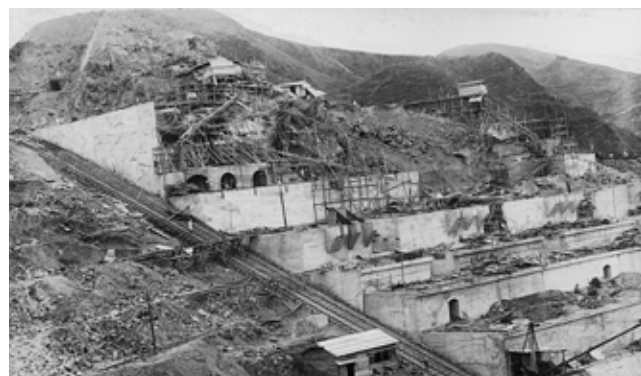
Smelter and refinery under construction
