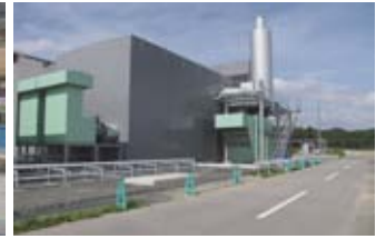
Private power generator (Isohara)
