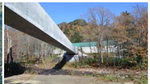
Bridge for water pipe and wastewater treatment plant
