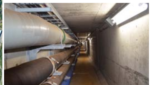
Inside a bridge for water pipe
