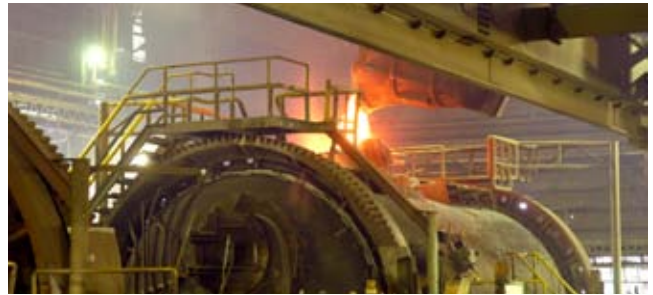
Anode furnace at Saganoseki Smelter & Refinery
