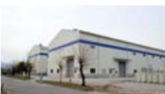
Building B for LiB Recycling at the Tsuruga Plant
