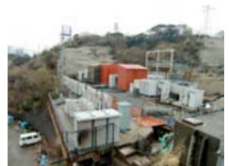
Secondary substation tentatively recovered by accommodating a feeder panel
