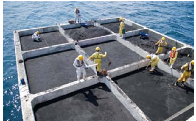
Caisson after iron silicate slag is dropped in
