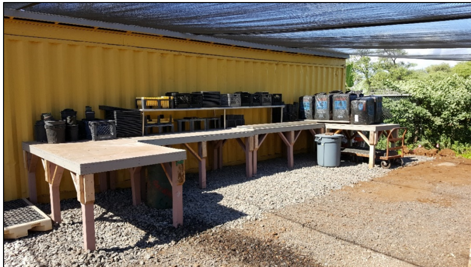
Figure 24 Weed cloth beneath coarse gravel under Kihei Nursery tables
