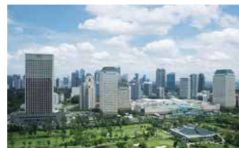
Senayan Square is a major development project comprising a shopping center, three office buildings, four apartment buildings, and a hotel complex. (Indonesia)
