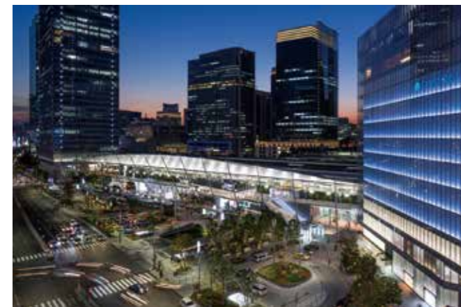
The redeveloped Yaesu side of Tokyo Station.
