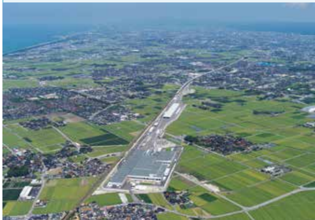
The Hakusan bullet train depot for the Hokuriku Shinkansen Line.
