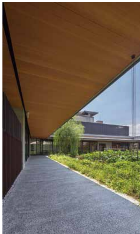
Kyoto Yaoichi Honkan, for which Kajima was honored at the 55th BCS Awards by the Japan Building Contractors Society.
