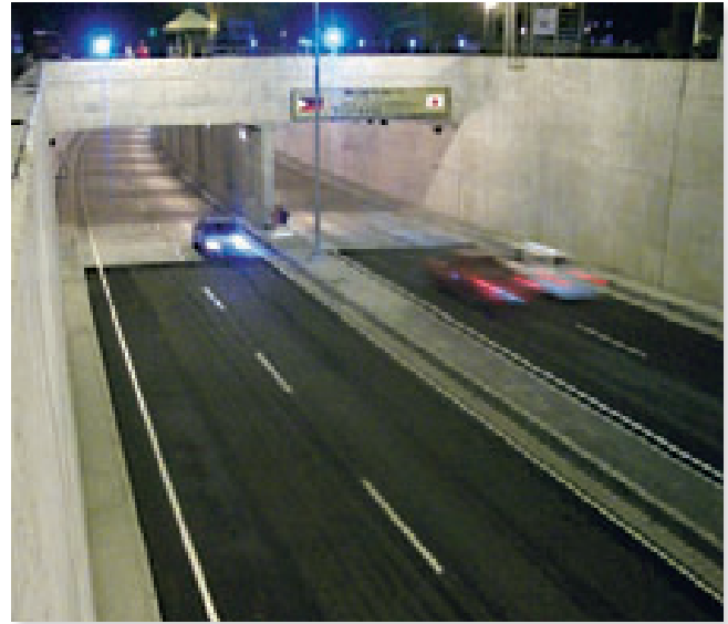
Cebu South Coastal Road, Philippines
