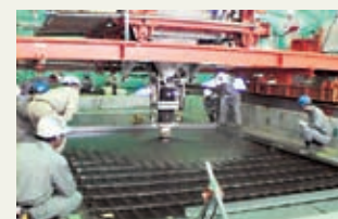
Test pouring of the concrete slab
