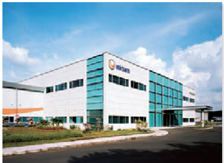
Unicharm No. 2 Indonesia Plant
