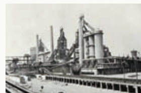
1962 Tobata Iron Mill, Yawata Iron and Steel Co., Ltd.
