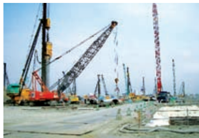
Steel pile construction work
