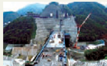
Casting the concrete body of the dam
