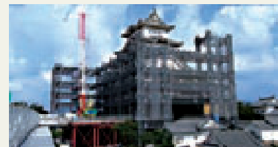
Himeji Castle under restoration
