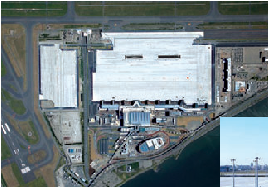
Tokyo International Airport (Haneda) International Apron
