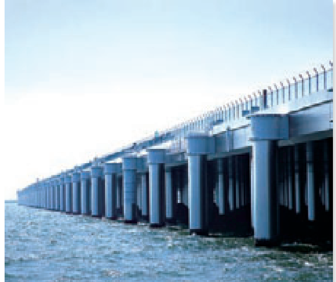
D-Runway of the Tokyo International Airport (Haneda)
