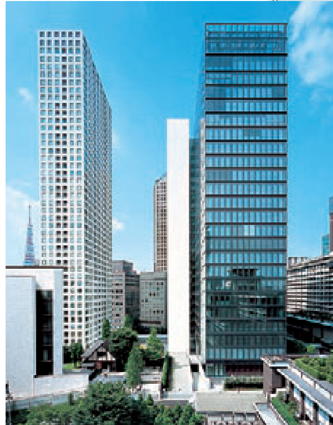
Toranomom Towers Office (Under operation since 2006)
