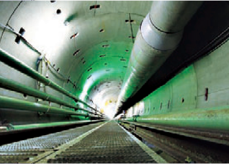
Shielded Tunnel for the Gas Pipelines across Ise Bay
