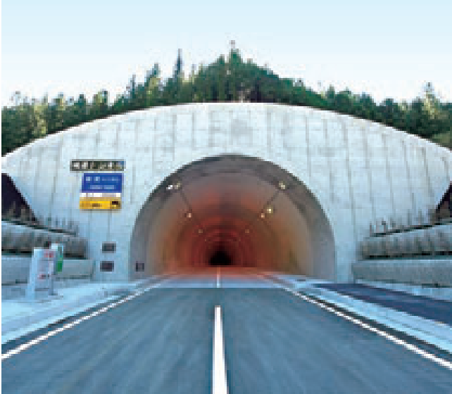
Jiyoshi Tunnel, National Highway No. 440
