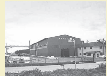
Hachinohe Office (now the Hachinohe Equipment Repair Center)
