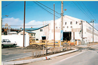
Tomakomai Sub-branch (now the Tomakomai Branch)
