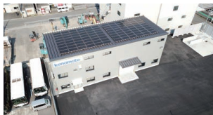
Solar Power Generation System Installed on the Roof of the Kyoto Branch Office
