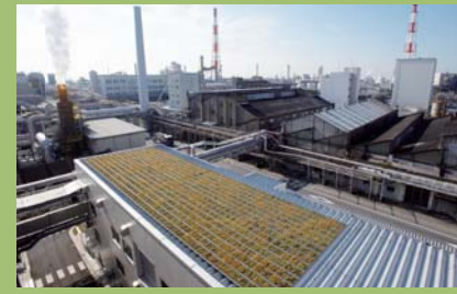
We grow vegetation on the rooftop of our Kanecaron plant
