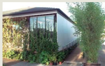
The green curtain cools the structure
