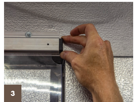
3 Secure strips with end caps.
