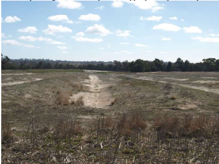
Photo 14. This ‘roaded catchment’ extending from crest unit C1 to upper slopes unit S1b is a water harvesting structure designed to increase the amount of surface runoff from the catchment above the largest dam near the central portion of Lot 52.
