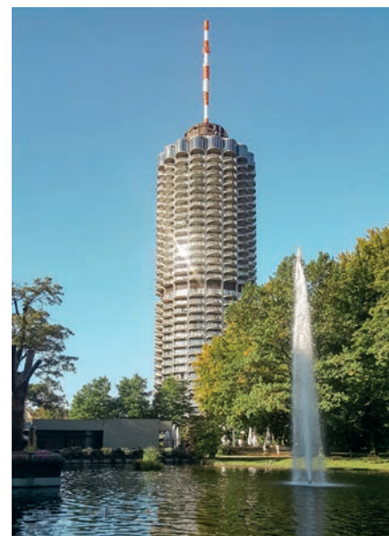
Outdoor monitoring and ANALYTICS Software in use at transmitting station "Augsburg-Hotelturnm", Germany
