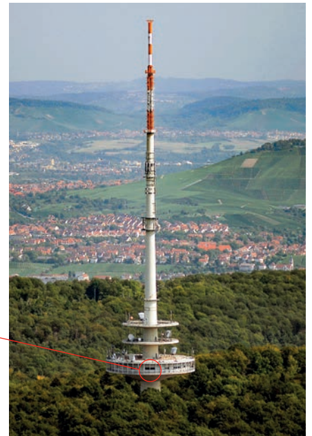
Indoor and outdoor monitoring implemented at FM transmitting antenna system "Stuttgart", Germany
