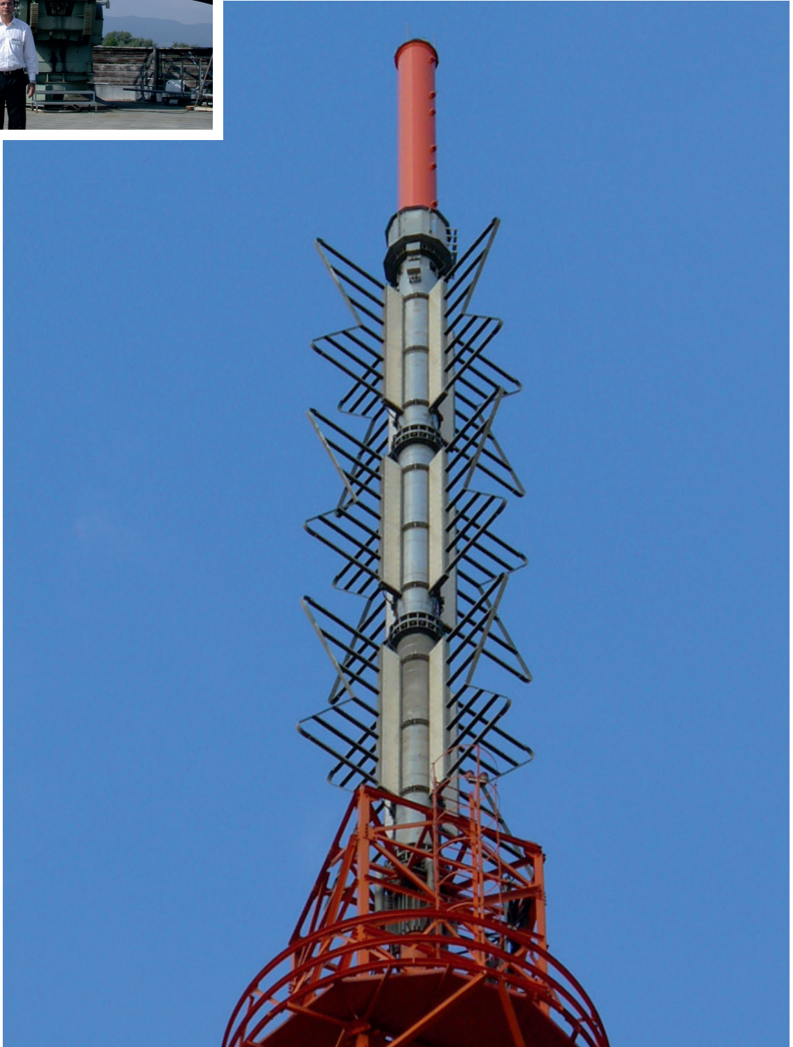
Superturndisk Antenna Station "Belo Horizonte", Brazil
