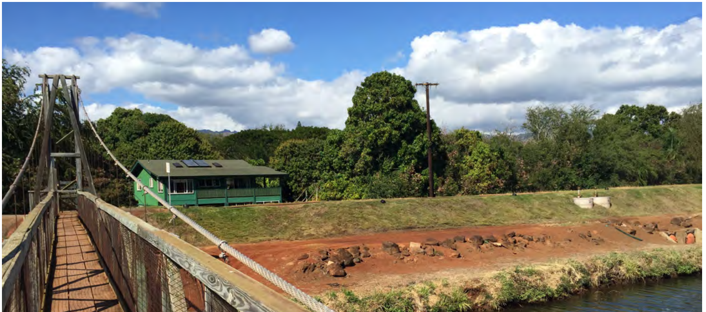
Historic Hanapēpē Swinging Bridge, Hanapēpē-'Ele'ele District
