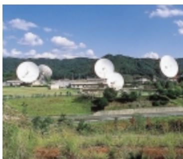
Yamaguchi Satellite Earth Station
