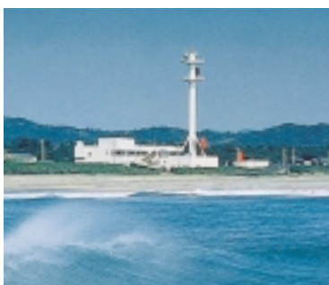
Chikura Cable Landing Station
