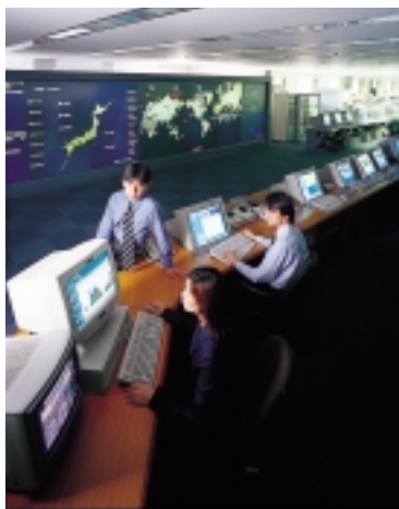
Network Center (KDDI Building, Shinjuku)
