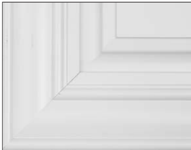
Example of front joint separation
