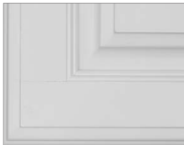
Example of front joint separation
