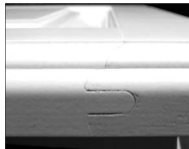
Example of end joint separation
