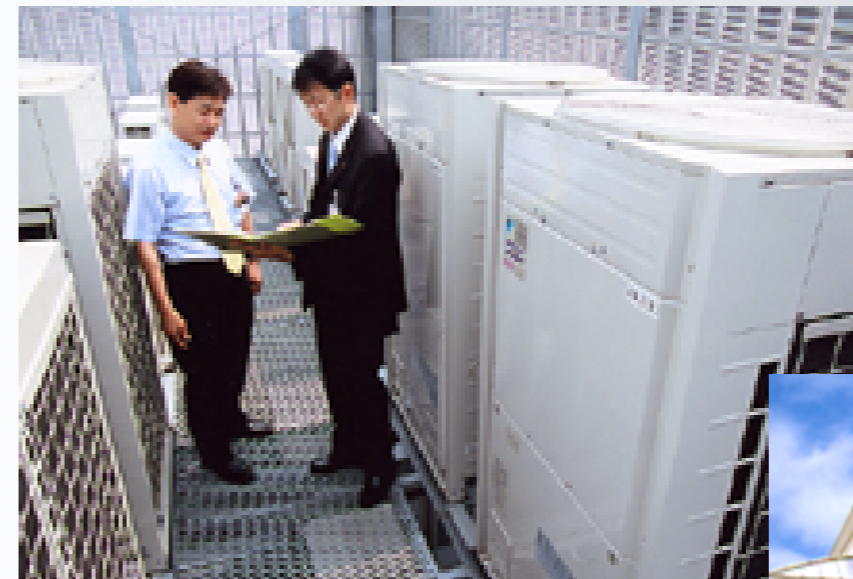
"Eco Ice" thermal storage system
