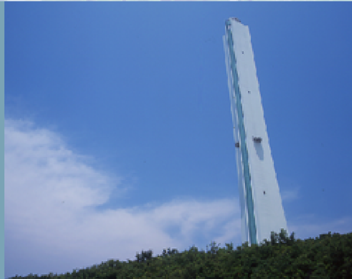
Nanko Power Plant (ISO14001 certified)
