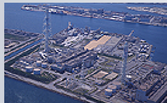
Himeji No.1 Thermal Power Plant
