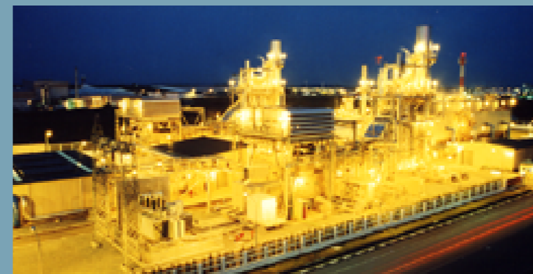
Thailand's Rojana Power Co., Ltd.
