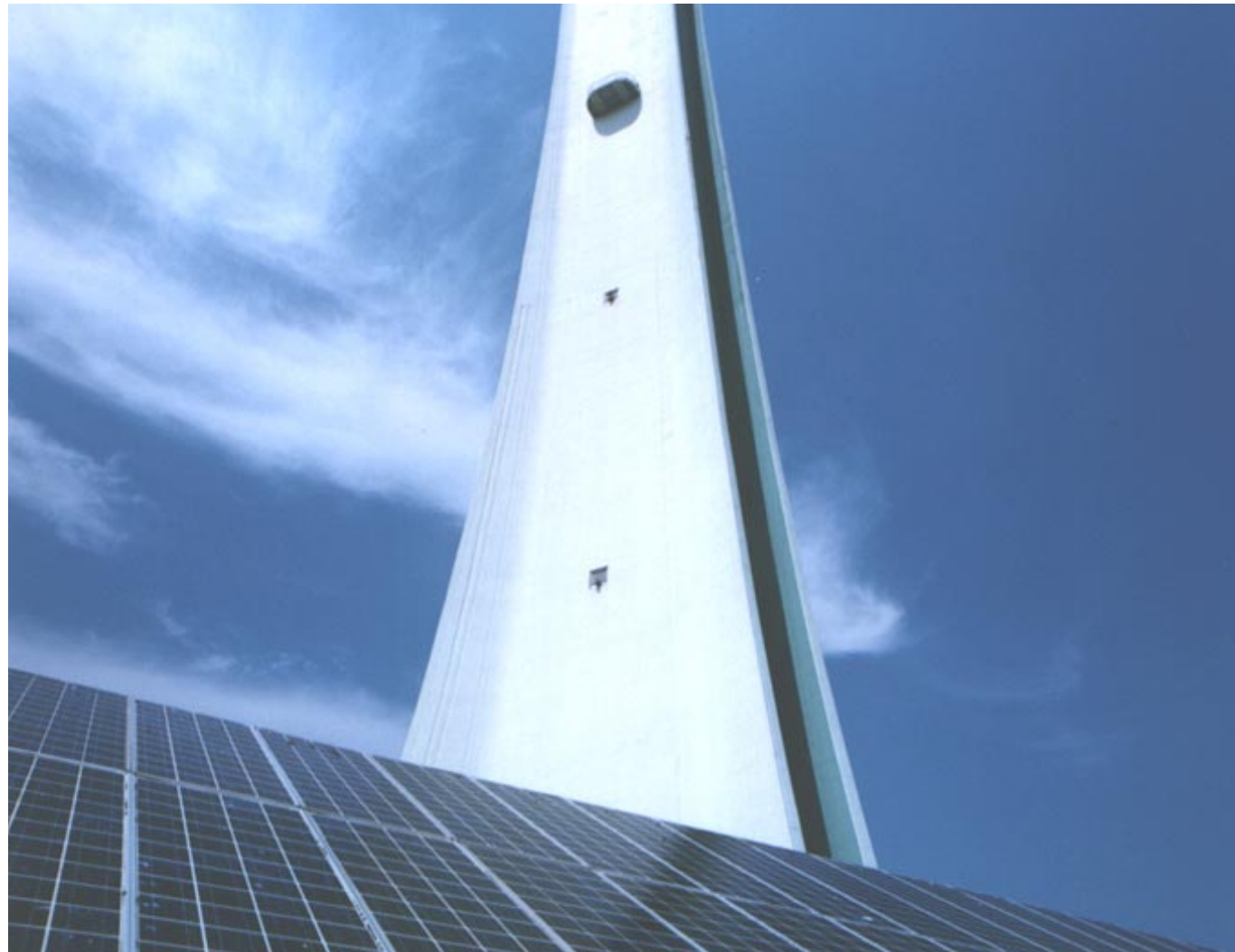
Photovoltaic power-generating devices and attractively designed flue (Nanko Plant)
