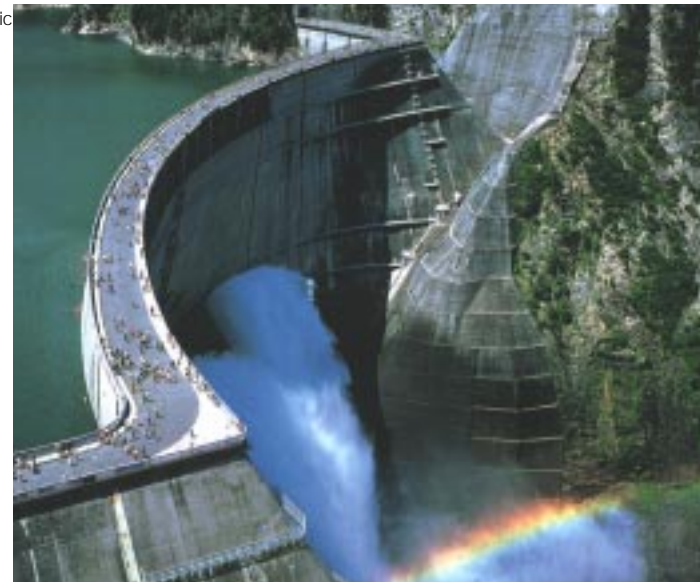
Kurobegawa No.4 Thermal Power Plant (335 MW)
