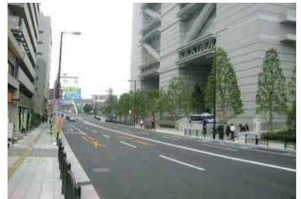
Underground power lines (The area around Osaka International Conference Center)
