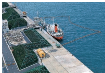
Oil fence at unloading dock
