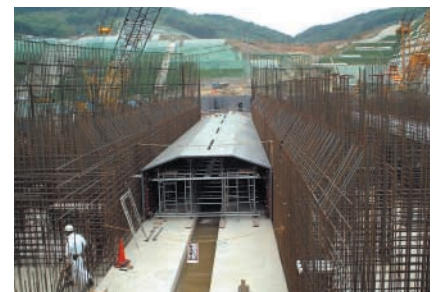
Metal frames used to erect a coal silo at the Maizuru power station
