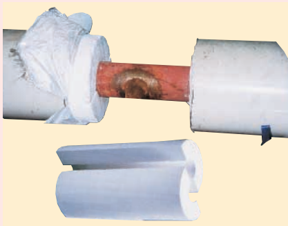
Insulation material for piping at power station
