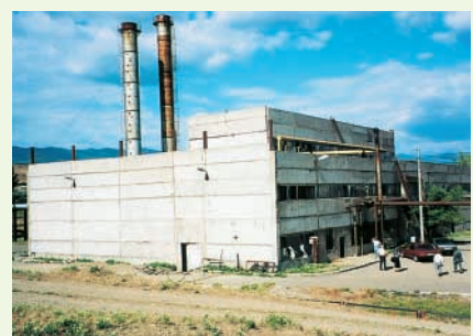
District Heating Plants in Tbilisi, Georgia
