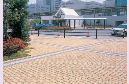
Seemingly warm walkway utilizing unbaked bricks (The area around JR Nishinomiya Station)
