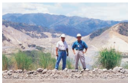
Construction site for San Roque Project
