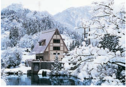
Sakaigawa Power Station
