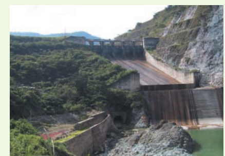
Binga Hydropower Plant (Benguet Province, Luzon Island)
