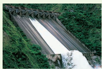
Ambuklao Hydropower Plant (Benguet Province, Luzon Island)
