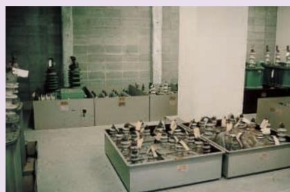
PCB waste storage facility
