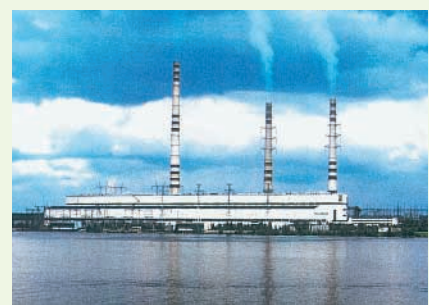
Konakovo Thermal Power Station (Moscow)
