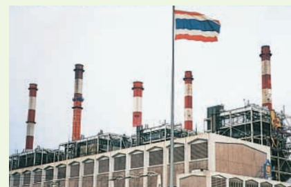
South Bangkok Power Station
