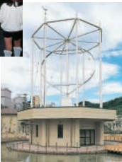
Darrieus wind turbine power generator
