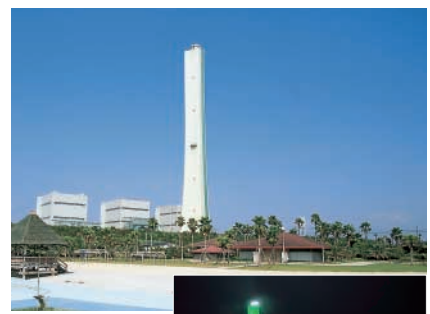
Nanko Power Station
