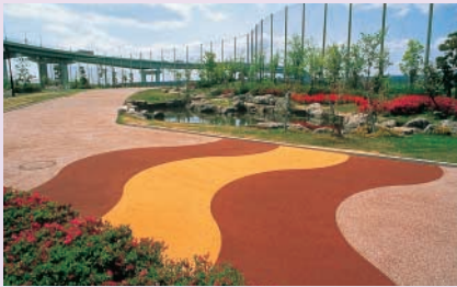
Water-permeable pavement from insulator scraps (Amagasaki Techno-land)
