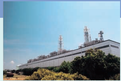
Himeji No. 2 Power Station
