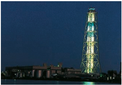
Himeji No. 1 Power Station
