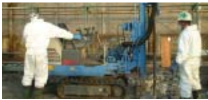
Soil testing by boring
