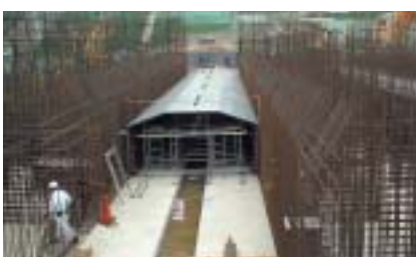
Metal frames used in the construction of the Maizuru Power Station
