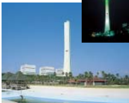
Designed as a monument, the smokestack at the Nanko Power station lights up different in each season.
