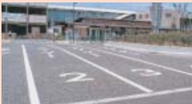
Bright-colored asphalt pavement in a parking lot
