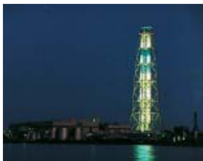
The smokestack of the Himeji No. 1 Power Station uses color-coded lights to report the tides, temperature and time.
