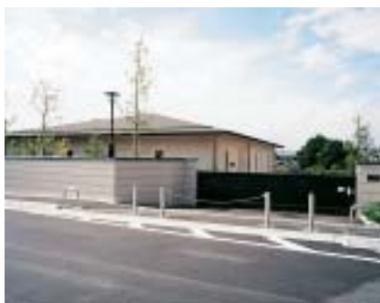
The Hoshida Substation was designed with a low roof to look like a home from the outside.
