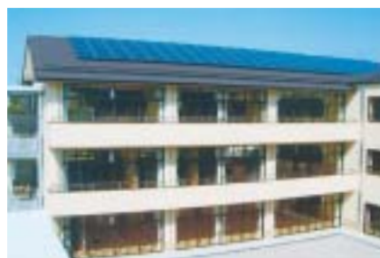
Solar panels on the Bandani Higashi Elementary School
