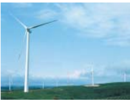
Sarakitomanai (Hokkaido) 1,650 kW X 9 units
