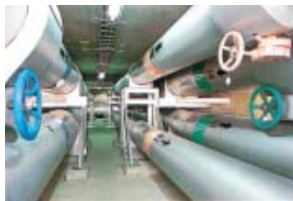
Utility tunnel and pipes
