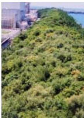
Ecologically planted area around the Gobo Power Station
