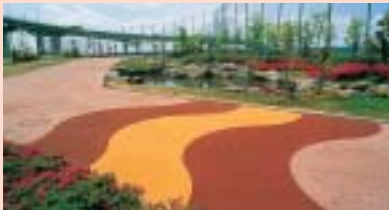
Water-permeable pavement at Amagasaki Techno-land
