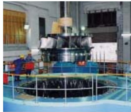
Replacement of a water turbine
