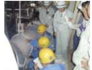
Inspection of secondary system piping using ultrasonic measurement
