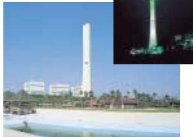
Designed as a monument, the smokestack at the Nanko Power Station lights up different each season.
