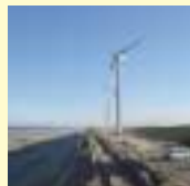
Wind power electricity generation equipment
