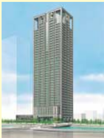
New Kansai Electric Building
