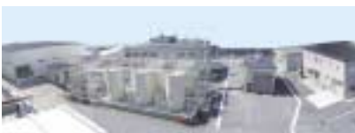
Recycle center for utility pole transformers
