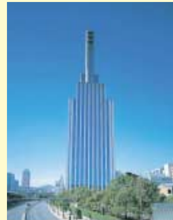
Kobe Kansai Electric Building
