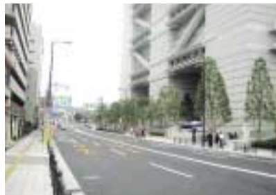
Power lines buried underground
