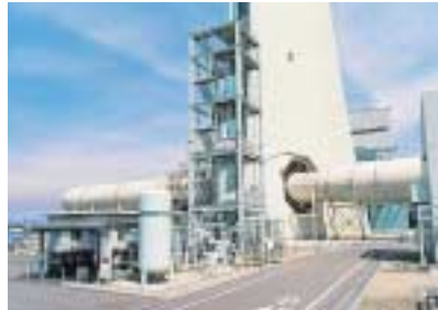
Flue gas CO 2 recovery pilot plant (Nanko Power Station)
