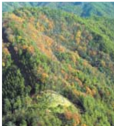
High voltage towers use minimal lighting in order to blend into the surroundings.
