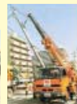
Electric wiring restoration
