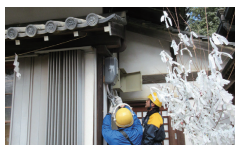
Inspecting electrical equipment at Sumiyoshi Shrine (Akashi City, Hyogo Prefecture)
