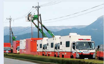
Our high-voltage generator vehicles supplying emergency power
