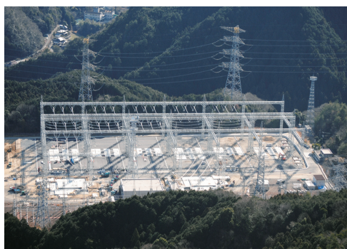
Construction of a new 500 kV substation
