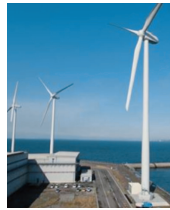
Tahara No. 4 Wind Power Station
