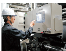
Inspecting the utility facilities of the Abeno Harukas building
