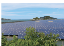
Arida Solar Power Station
