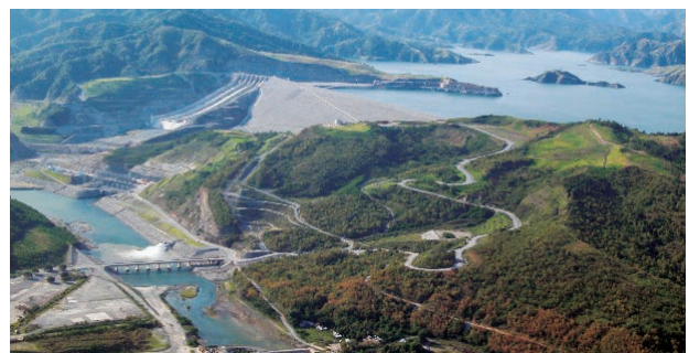
View of the San Roque Hydropower Station in the Republic of the Philippines
