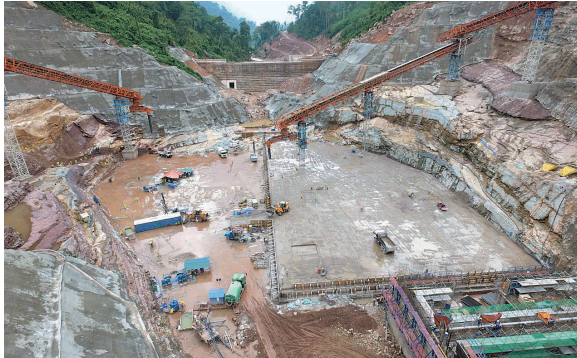
Dam construction site
