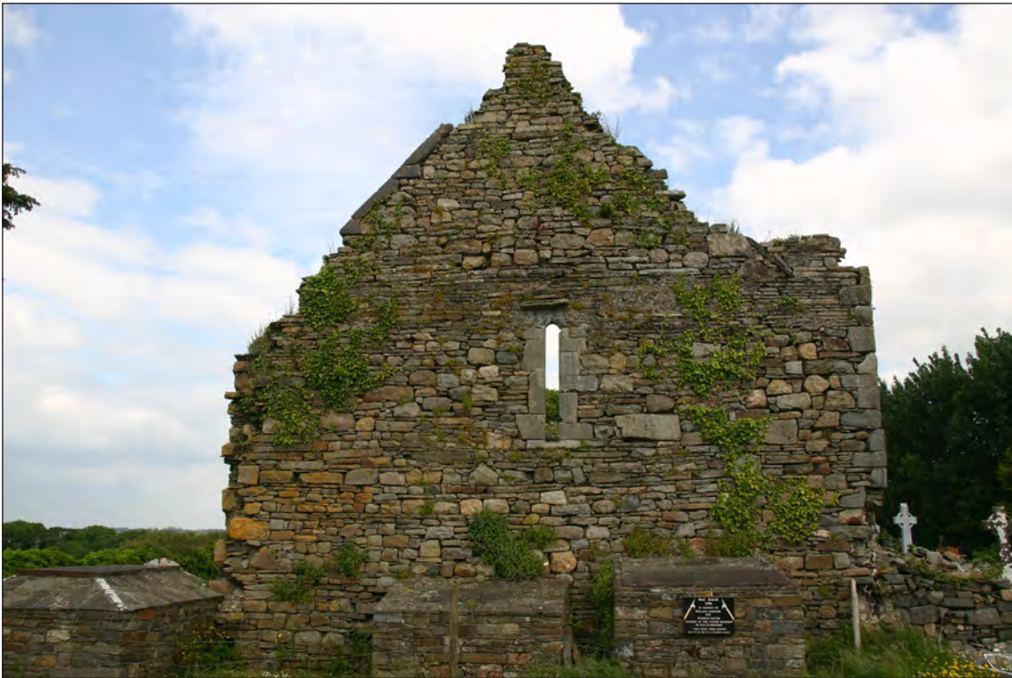
Plate 13: View of the exterior west gable of Aghavallen Church. Note lean-to tombs and robbed out quoins. Further note projecting drip stone over window and surviving cut stone coping on gable as well as surviving gable shoulder on right (south)
