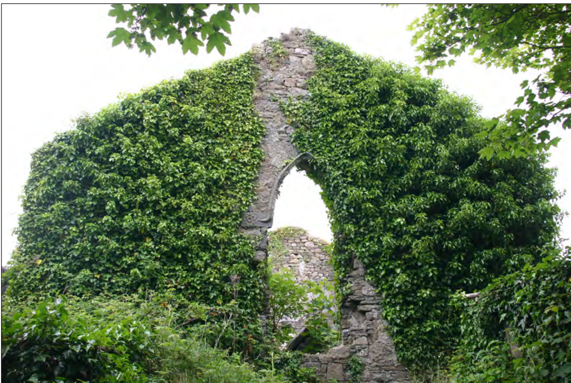
Plate 28: View of the exterior, overgrown east gable of Aghavallen Church. Note large central window, largely robbed out but still retaining sections of its dressed masonry including its hood moulding
