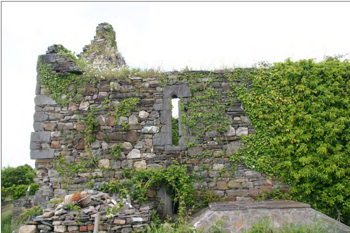
Plate 30: View of western limits of south elevation. Note upper and lower windows. Further note remains of gable shoulder, robbed out lower quoins and overgrown walls
