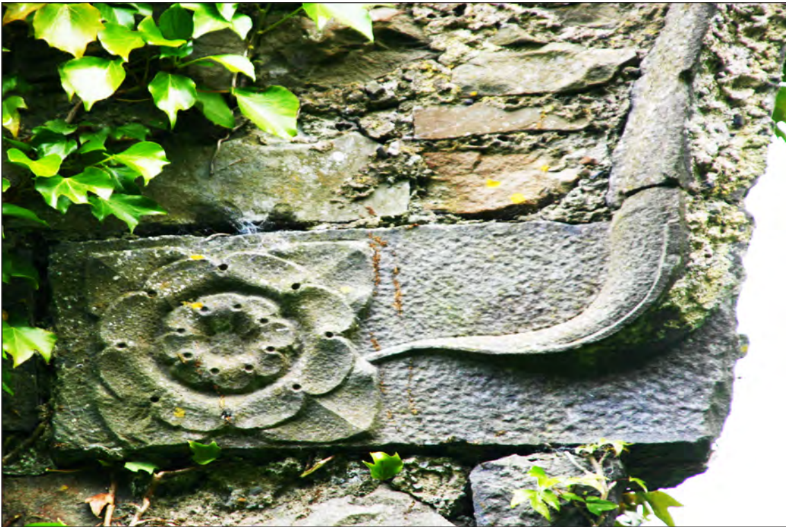
Plate 29: Close up view of rose motif detail on terminal of hood moulding over exterior of east window
