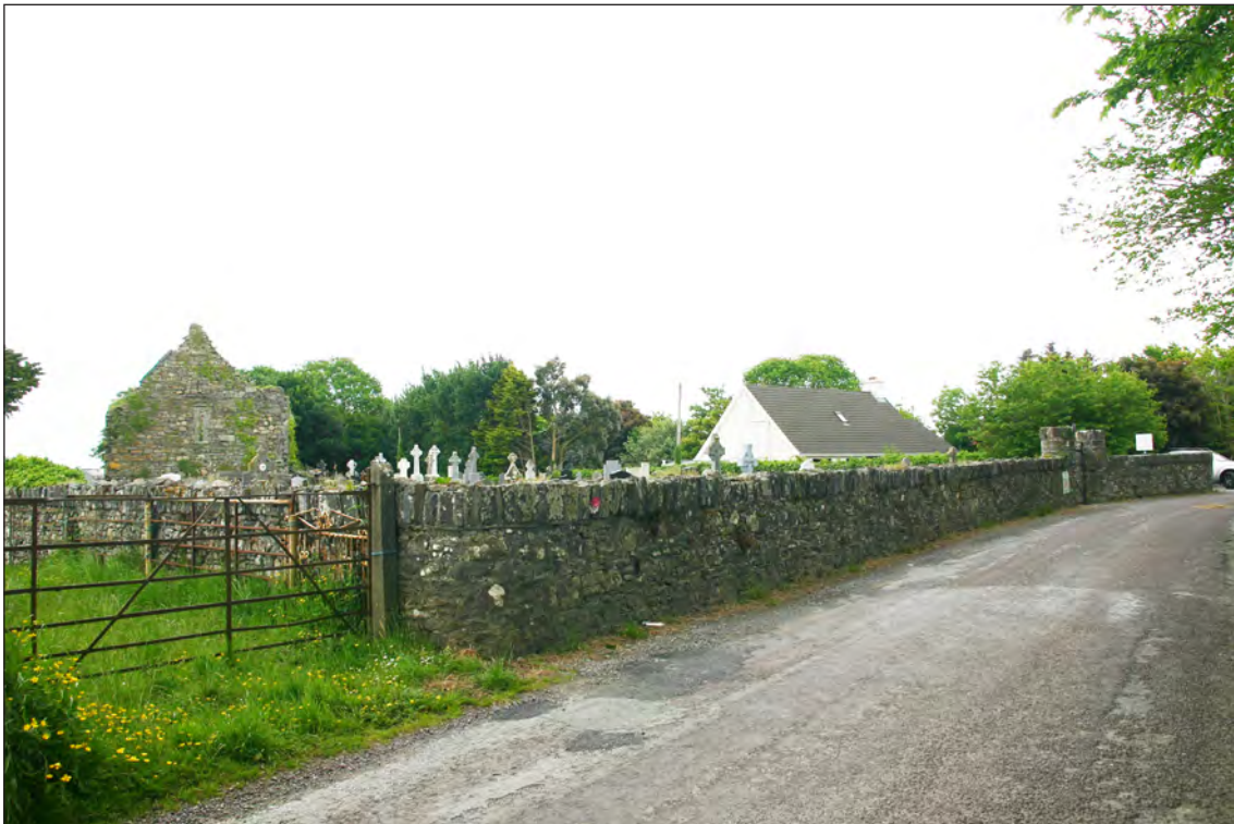
Plate 4: View of Aghavallen Church, Graveyard and boundary wall, from the northern approach
