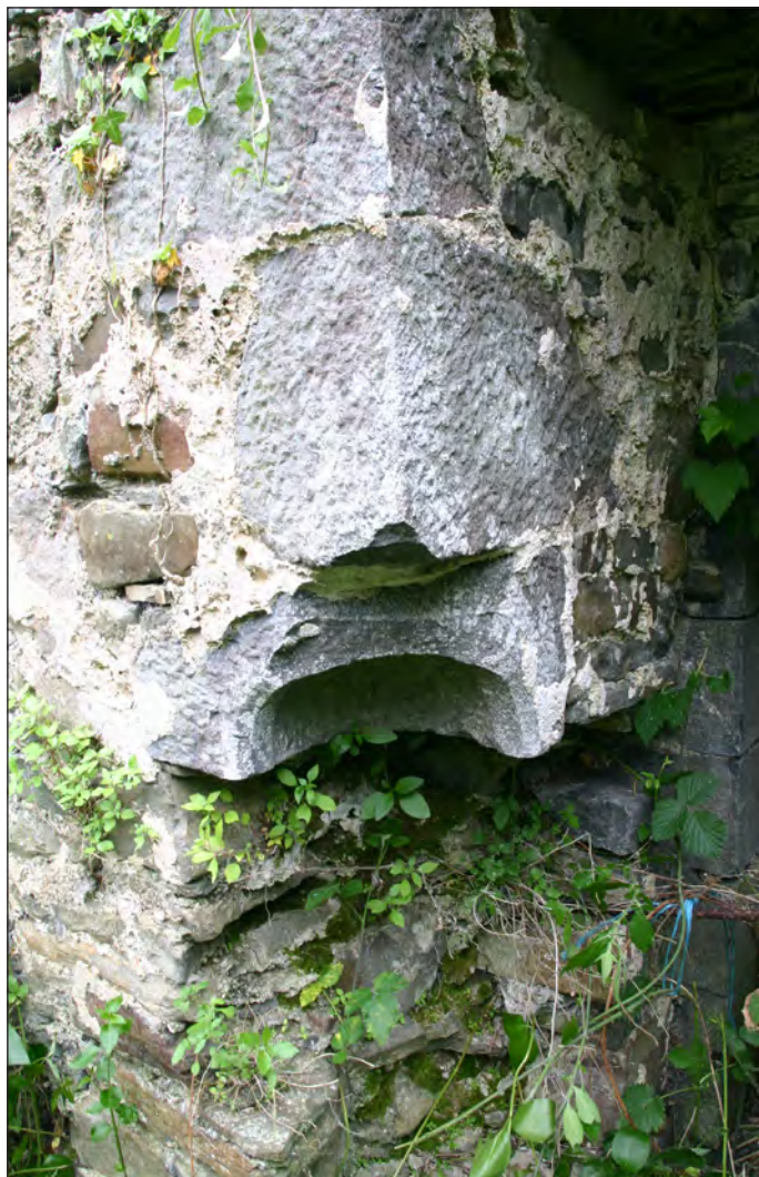
Plate 32: Close-up view of partially destroyed, possibly double entry, stoup on inside east side of doorway on south elevation
