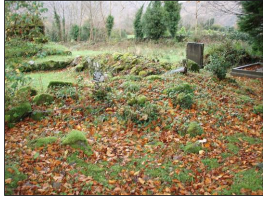
Pl. 8. Rubble collapse at N and W walls of church
