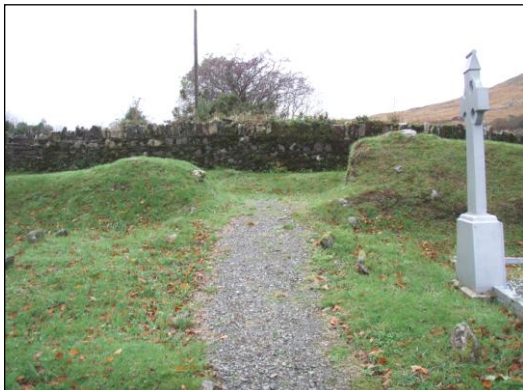
Pl. 3. Breach in bank on N side
