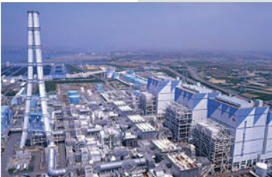
Flue gas desulfurization plant for Chubu Electric Power Co., Inc.
