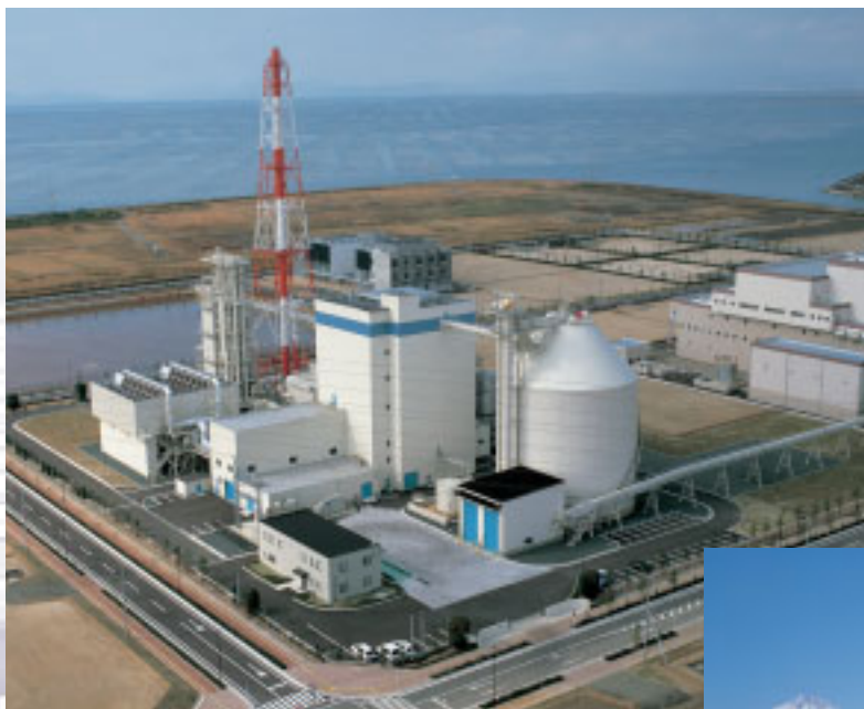
▲ Refuse-derived fuel power generation plant for Omuta Recycle Power Co., Ltd.
