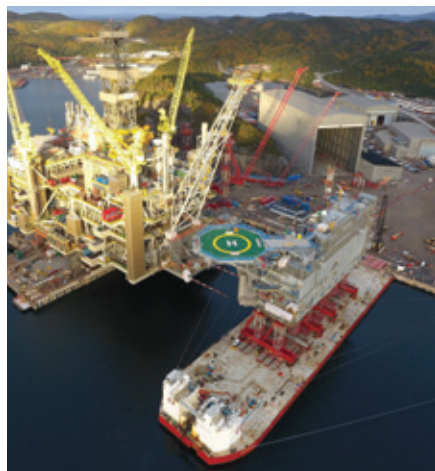
The LQ module was loaded onto the barge.
