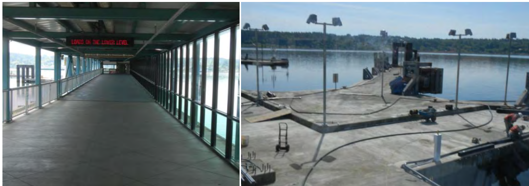
Figure 5-2: Existing Bremerton POF Facilities (Float B Covered Walkway pictured left and Float A under construction pictured right)
