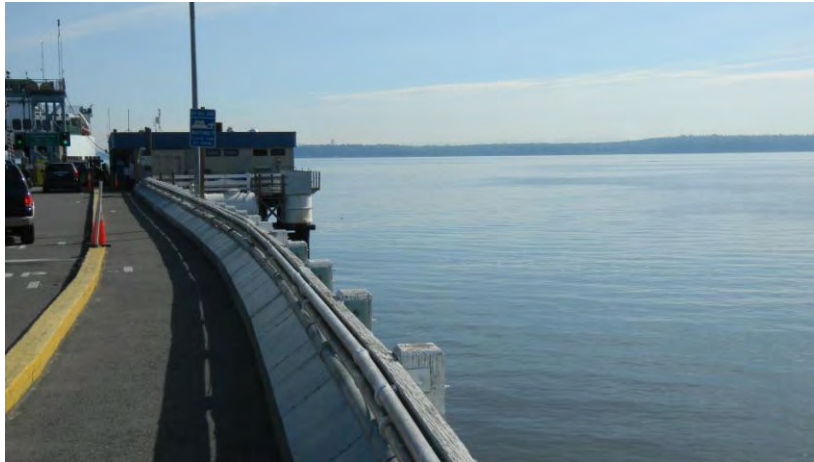
Figure 5-6: Existing Pedestrian Pathway and terminal building on WSF trestle at Southworth
