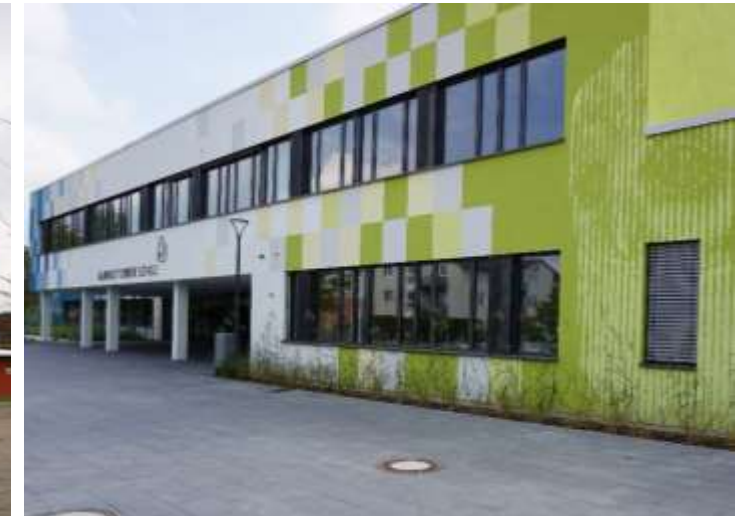
New fassade with tripple glazed wood-aluminium windows in PH-quality ( U_w \sim 0,8 \text{ W}/\text{m}^2\text{K} )
