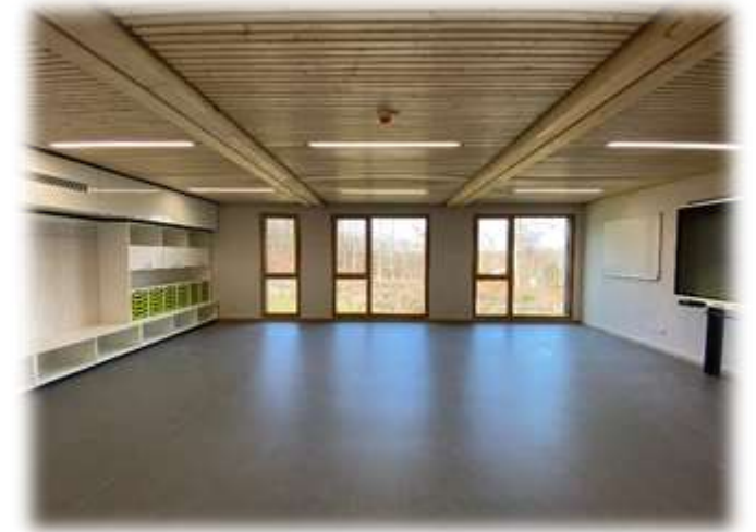
Class room with integrated ventilation unit in furnitures at left side
