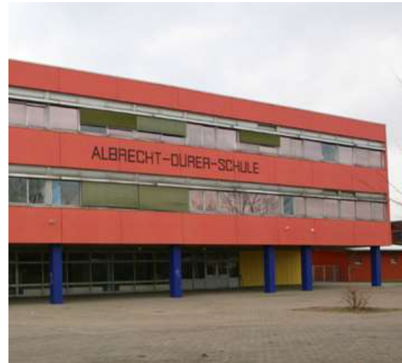
Old fassade with baldy insulated aluminium windows
