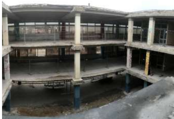
Construction: dismantling of the whole building and reconstruction
