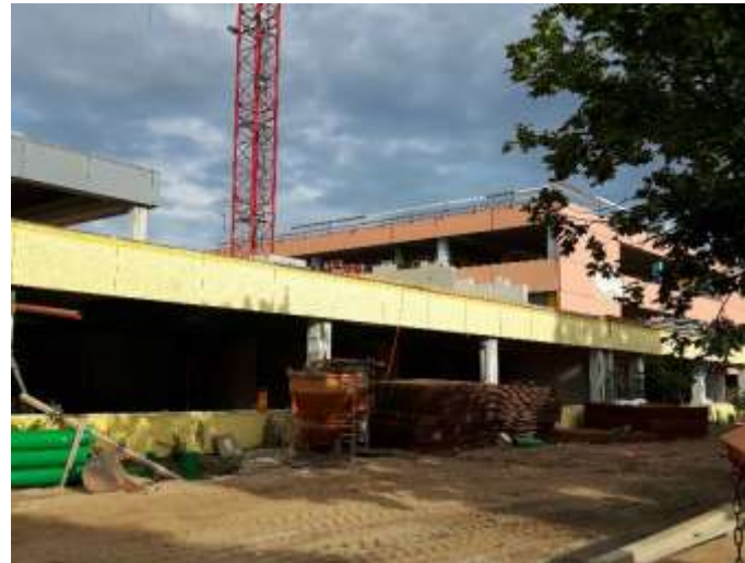
Outer view during construction
