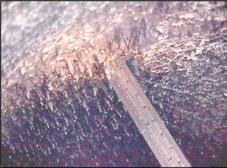
Polymer laced inlet pipeline
