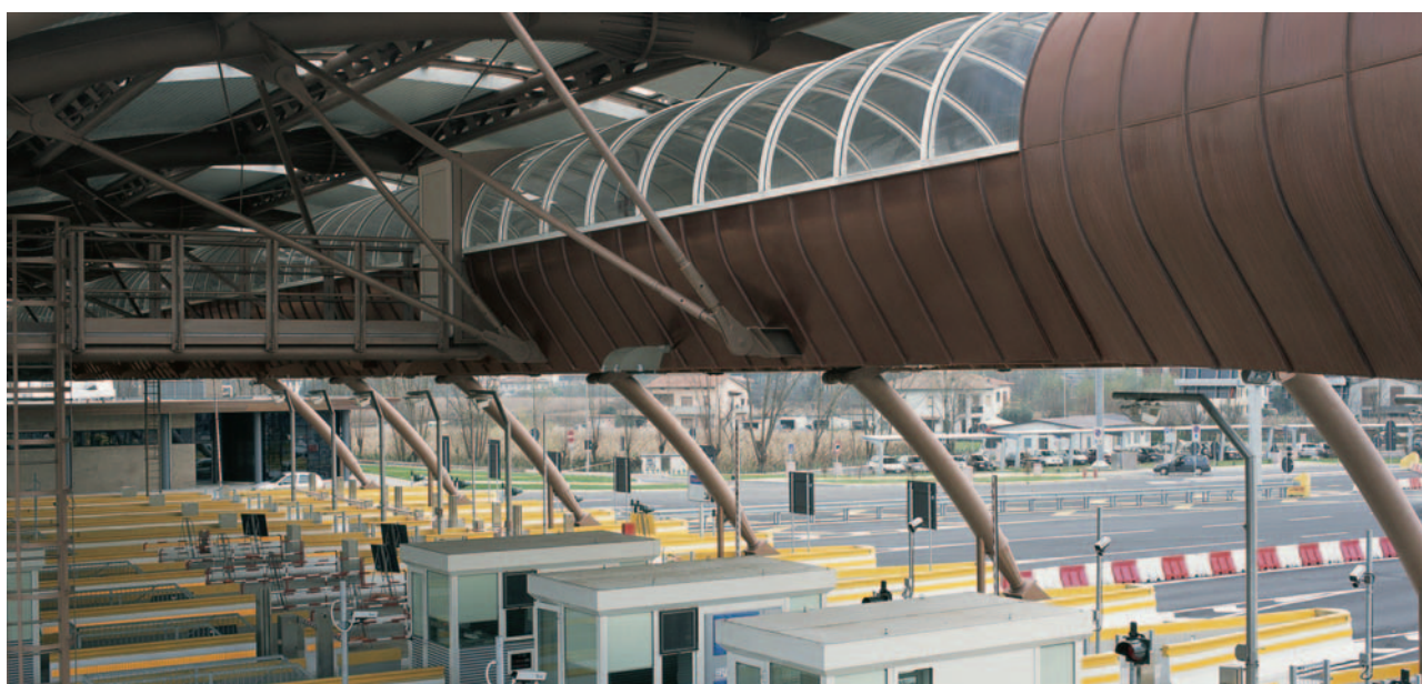
Coating in Tecu® Oxid – Motorway tollgate at Lucca.
