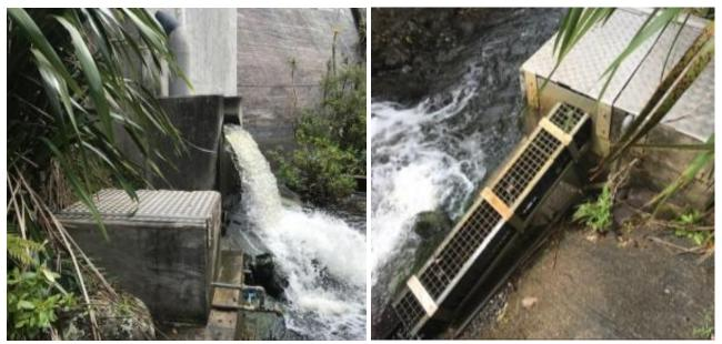
**Image on left:** Waitākere Dam trap location (Waitākere compensation flow release point). **Image on right:** Waitākere Dam trap (fish path and trap).
