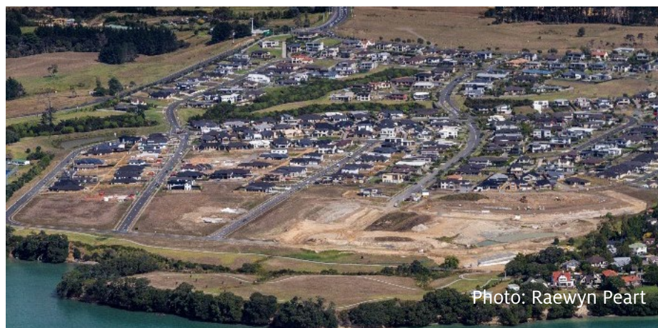
Figure 7.8 Large scale earthworks for residential development
