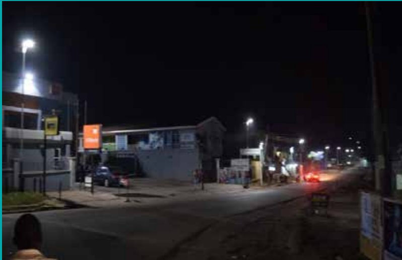
Streetlight Installation from GTbank to NTA roundabout
