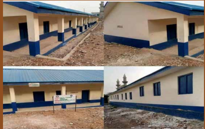
MAHDI LGEA Primary School after Renovation
