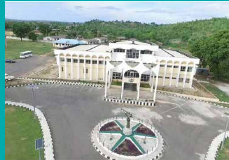
Kogi State House of Assembly Complex
