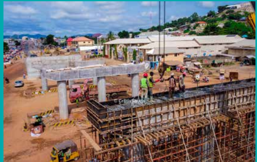
Ongoing Construction of Ganaja Flyover Bridge Lokoja
