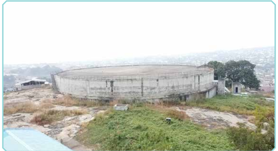
Lokoja City Water Works
