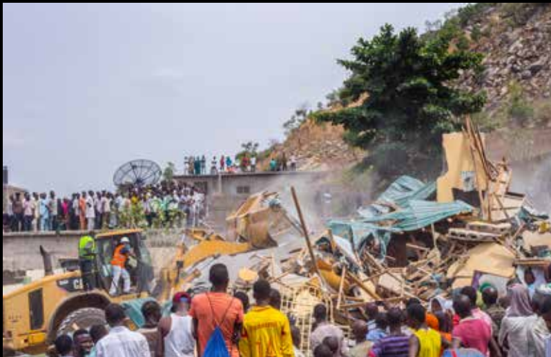
Demolition of Criminal Hideouts
