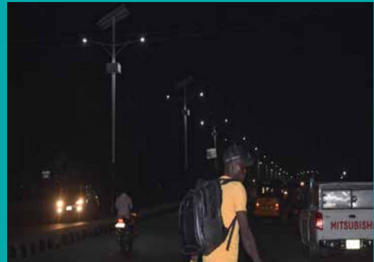
Installation of 1,300 streetlight pole from Nataco to Zone 8
