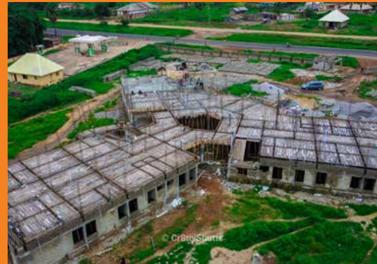
Ongoing construction of Ultramodern General Hospital Complex Eganyi
