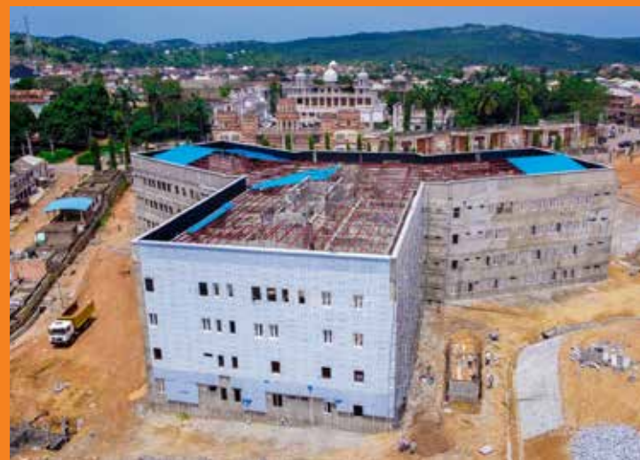
Ongoing construction of the Reference Hospital Okene
