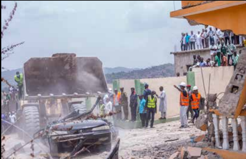
Demolition of Criminal Hideouts
