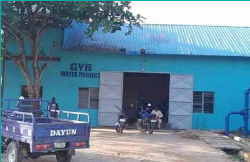
Okene Mega Water works
