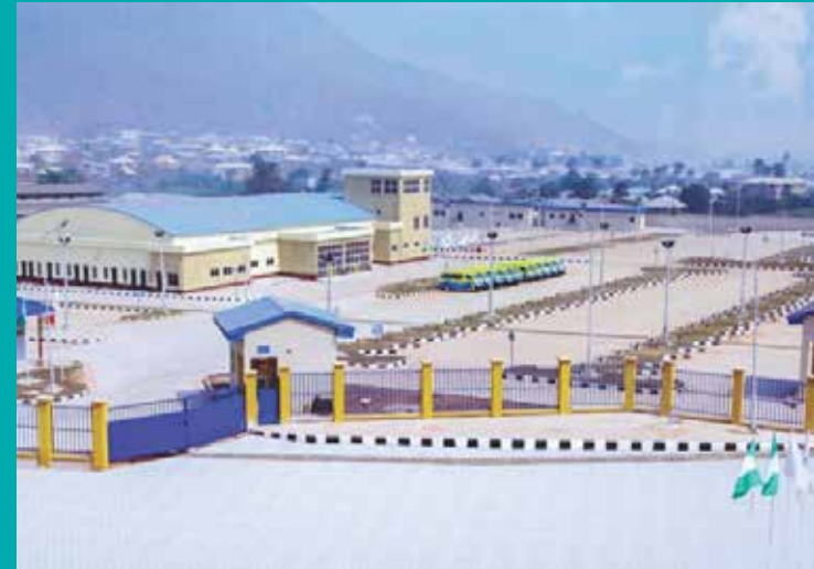
Completed Lokoja Bus Terminal
