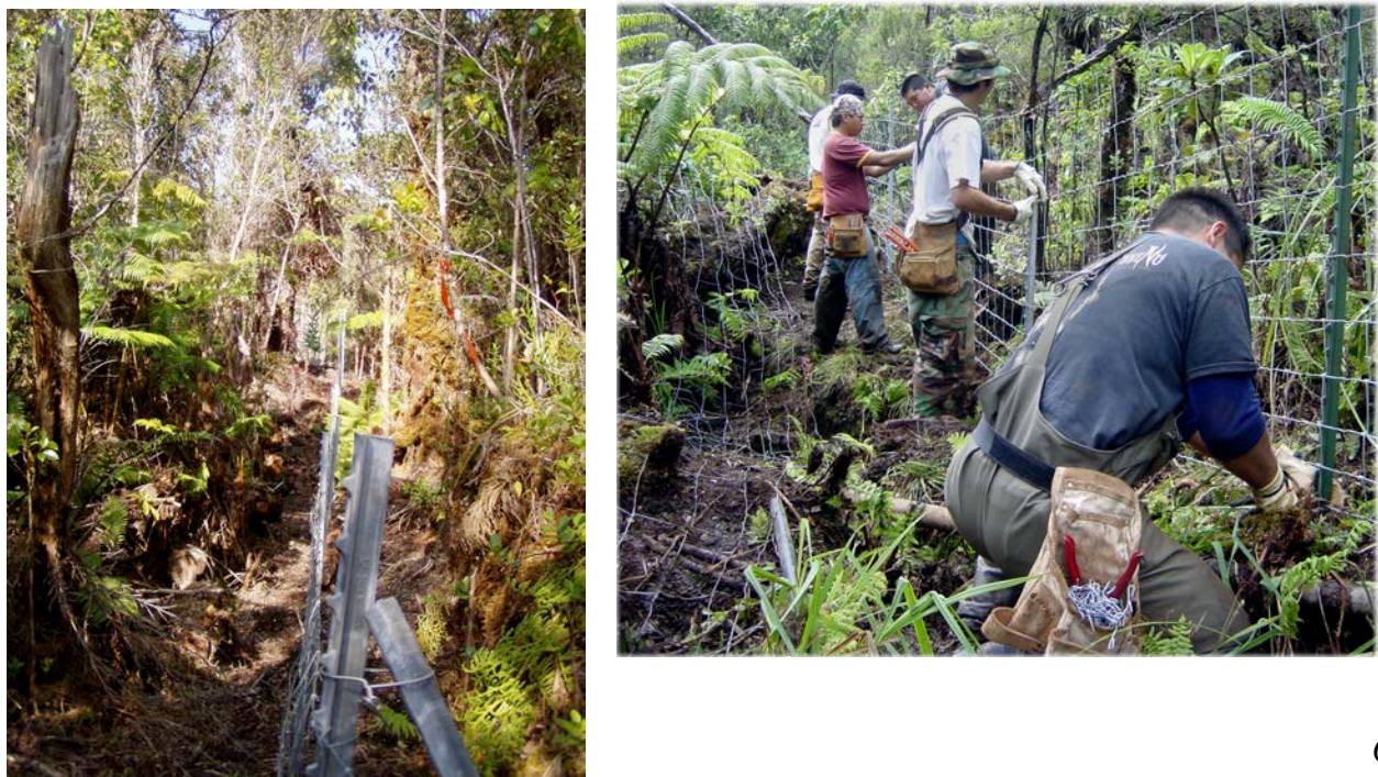
Photo 2: Fence construction projects on Maui and Hawai‘i.
