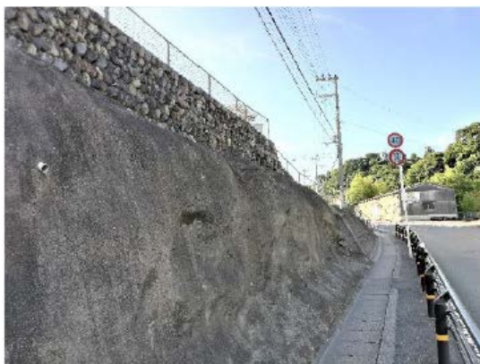
Fig. 14 A concrete retaining wall along a road [11]
