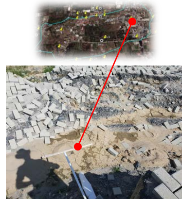
Fig.5 One of sand boil at Lolu Village site
