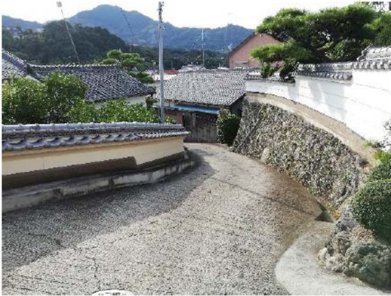
Fig. 7 Japanese style walls on the stone retaining walls [11]
