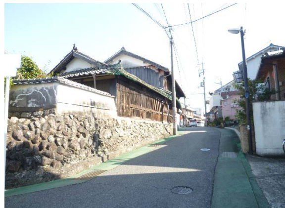
Fig.11 A stone retaining wall as a foundation for a traditional house
