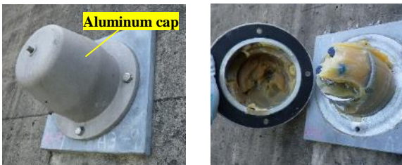
(b) Filled with corrosion inhibitor
