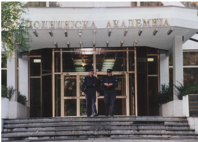
ENTRANCE TO THE BUILDING OF THE POLICE ACADEMY - IN BANJICA, BELGRADE. (THE BUILDING WAS DESTROYED IN THE BOMBING OF 1999)
