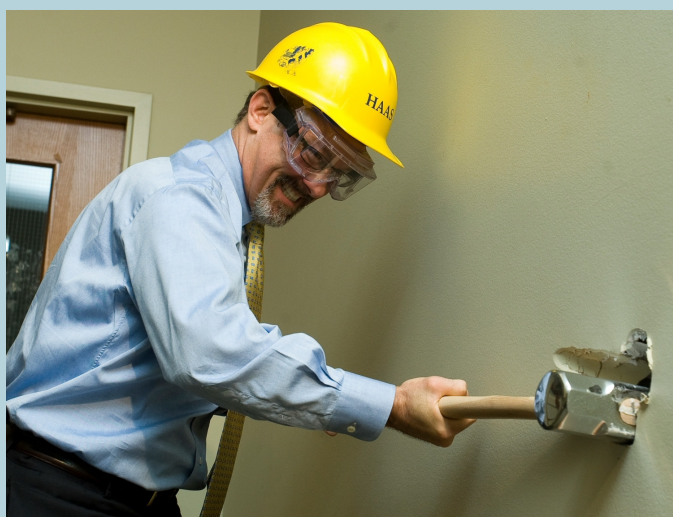
Dean Rich Lyons gets construction underway on the new high-tech classroom.
