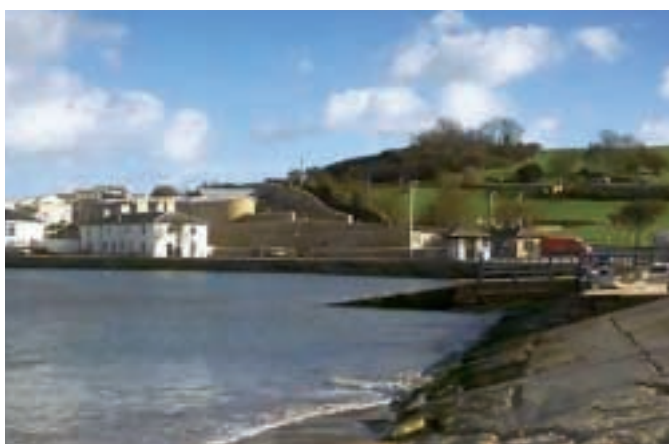
Our submerged membrane units have been adopted in the European countries. Photo: Swanage wastewater treatment plant in England adopting the submerged membrane units
