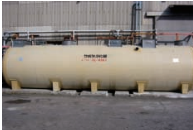
Joukaso installed in a hotel in Saga Prefecture K-HC-R2: 436 people, 88 m 3 /day (flow control tank + concentrated sludge tank)
