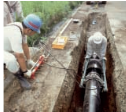
NS quake-resistant joint parts of ductile iron pipes
