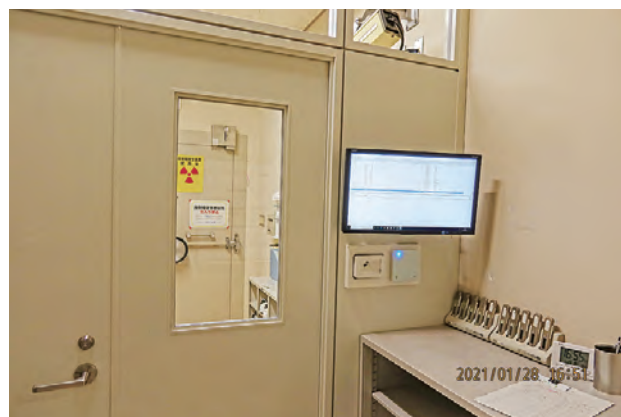
Figure 2. Renewed Entrance and Exit Management System.
