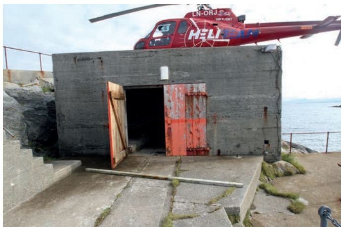
Over: Betongnaustet, fasade mot vest.
