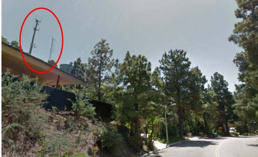
View 2: Looking East from 1896 Loma Vista Drive, Beverly Hills, CA
