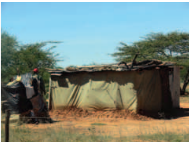
Corrugated iron sheeting as a roof with military canvas for walls, 5 February 2010
