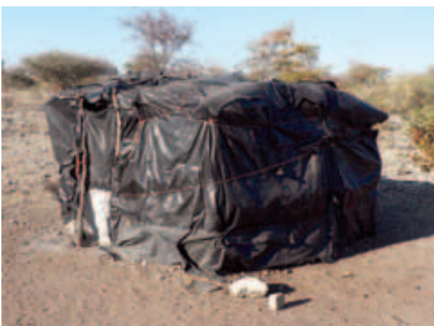
Black plastic sheeting for the entire structure, 13 July 2010
