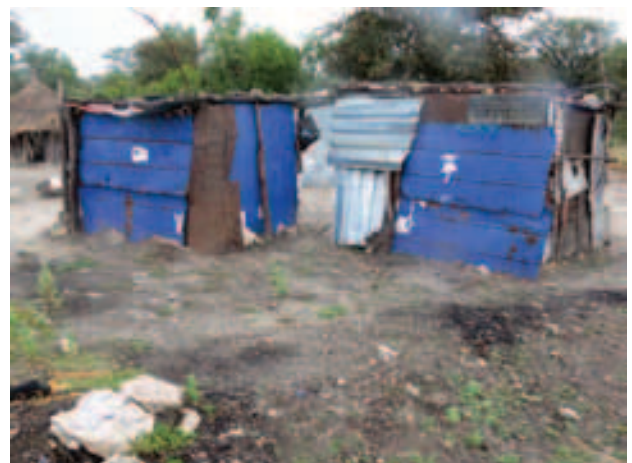
Corrugated iron sheeting as a roof and for walls, 26 March 2010
