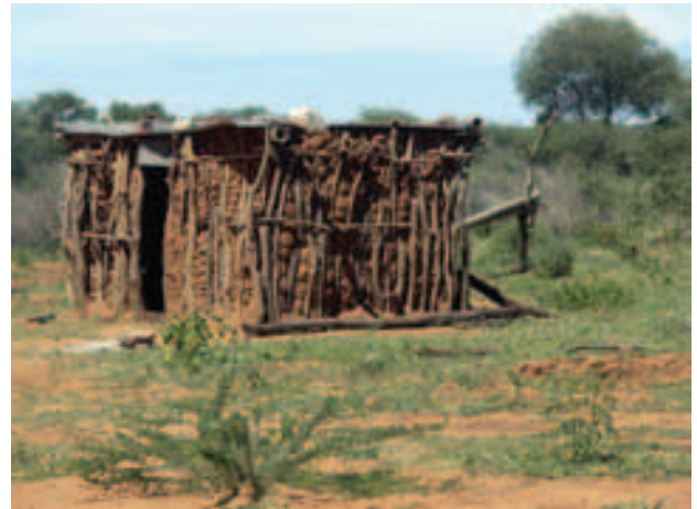
Traditional dwelling with corrugated iron sheeting as a roof, 2 February 2010
