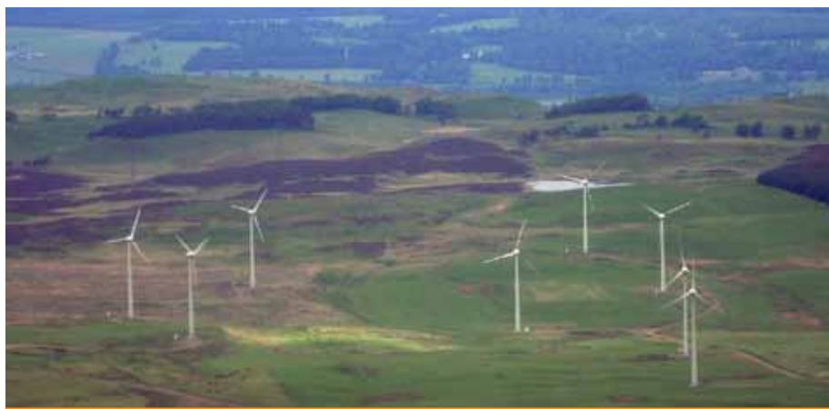
An on-shore Scottish wind farm
